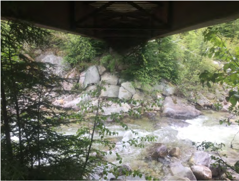
Left Bank Abutment when facing downstream
