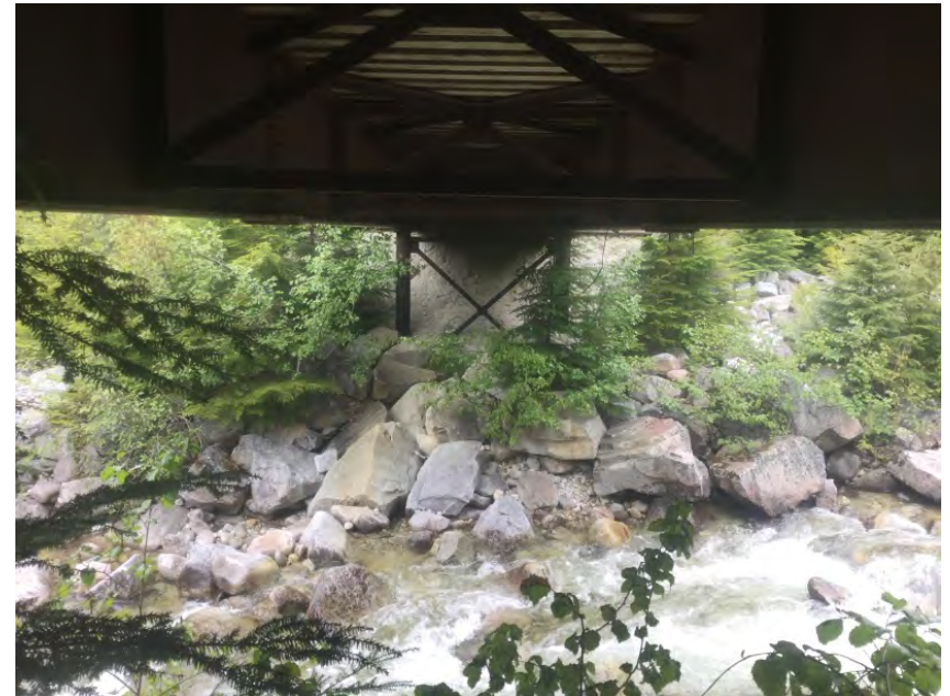
Right Bank Abutment when facing downstream
