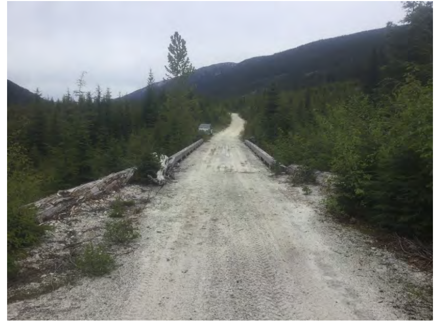
Approach from Left Bank when facing downstream
